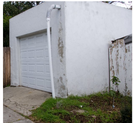
An example of what can be done with a down-spout; route the water into a planted basin, in this case, a young fig tree. Photo by Fang Lui
